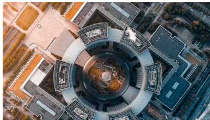
1.2MW ☰ Hangzhou Civic Center Podium Roof Photovoltaic Power Station 📍 Hangzhou, Zhejiang Province, China
