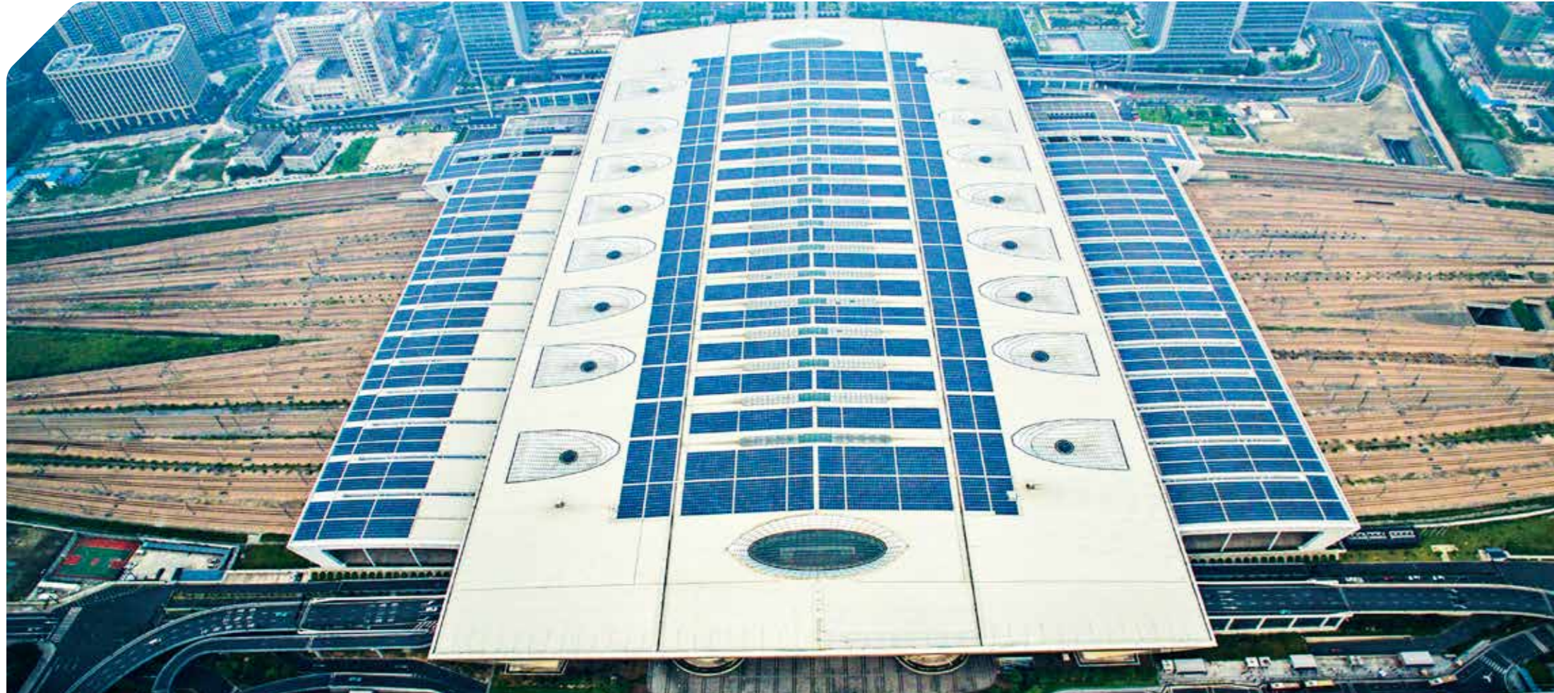
10MW ☰ Roof Photovoltaic Power Station of Hangzhou East Railway Station 📍 Hangzhou, Zhejiang Province, China
