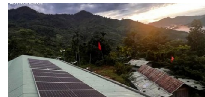
Vietnam PV Donation Project
